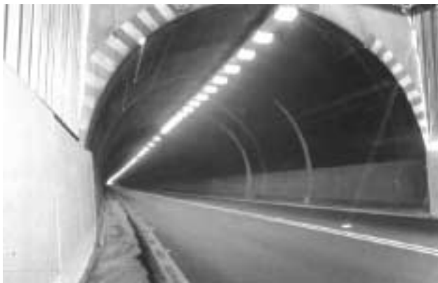
Figure 2 | PV lighting of tunnel no. 9
